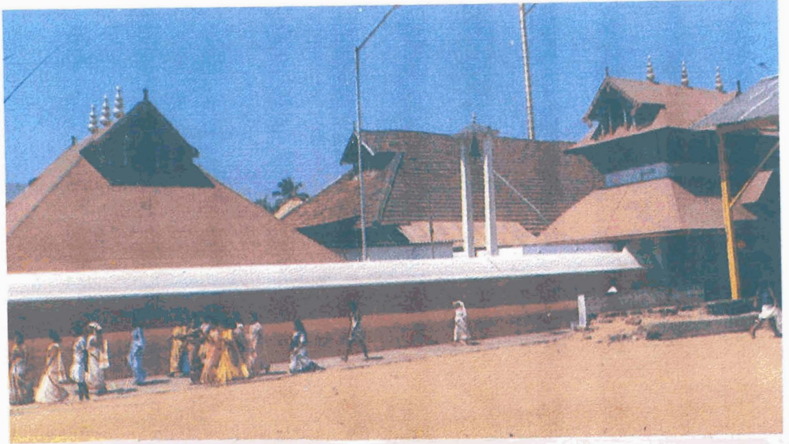
View of the Guruvayur Temple From South East
