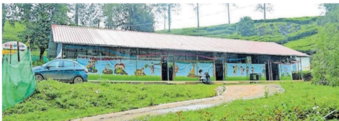
Fig. 5.16 Temporary School Building (Puthumala Govt LP School Building)
