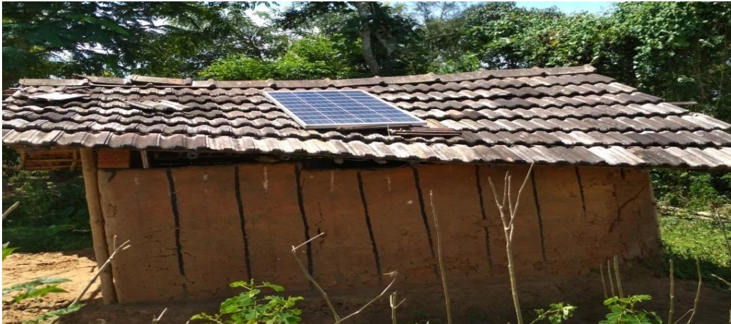
Solar panel construction in Kattunaykkan tribal communities in Wayanad
