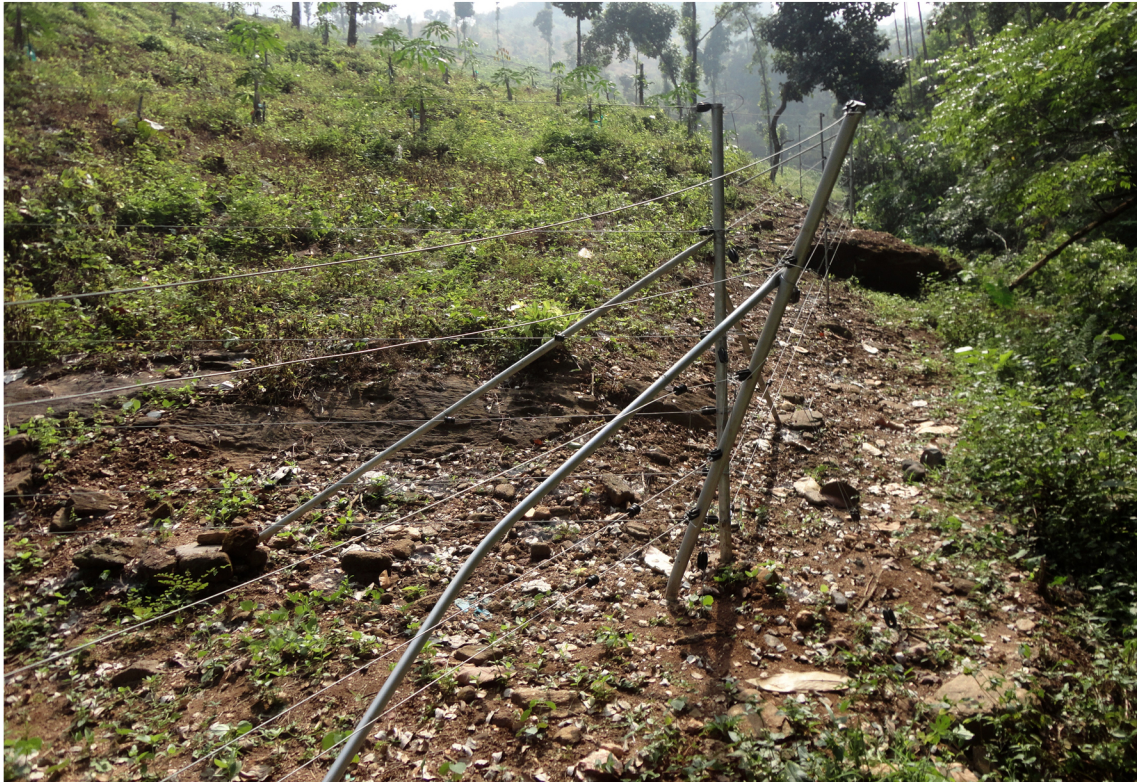
a. Solar electric fence damaged by Asian elephant at Karuvarakundu (Kalikavu Forest Range)
