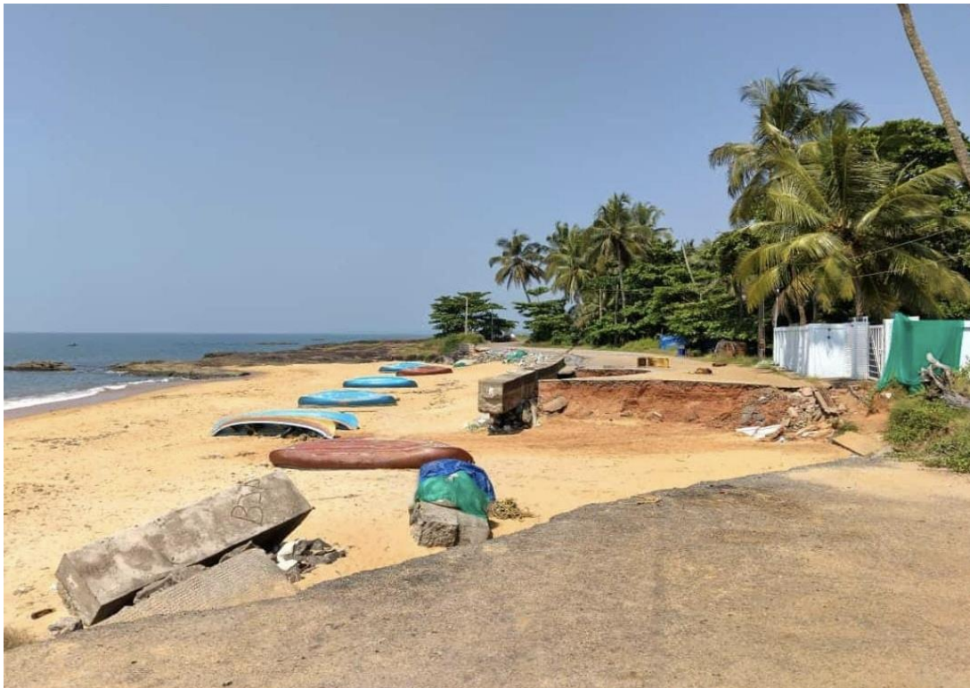
Coastal Road Near Ariyallur Damaged in Sea Erosion, Personal Collection
