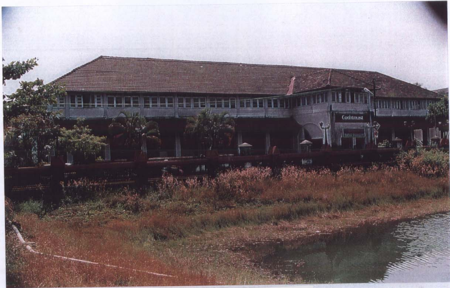
6. COMMONWEALTH TRUST INDIA (LTD) CALICUT (Front View)
