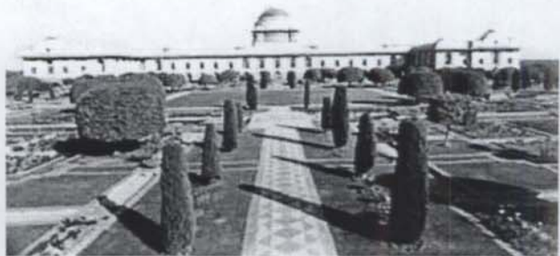
Figure 4.14 Rashtrapati Bhavan Gardens A view from south
