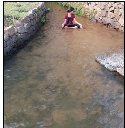
5 (102). Irrigation canal (Maneed)
