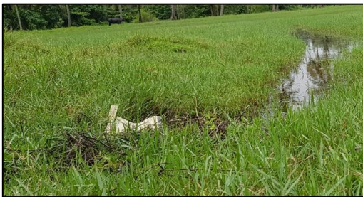
5 (167). Ditch in abandoned paddy field (Karingachira)
