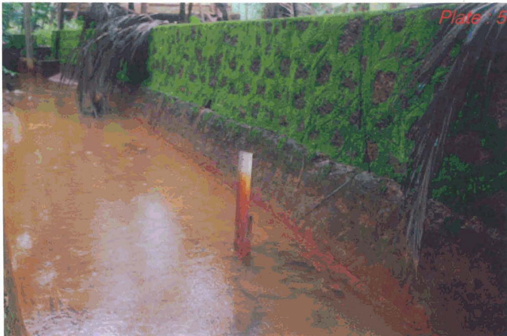
Plate : 4 & 5 Discharge of mine effluents through natural drains
