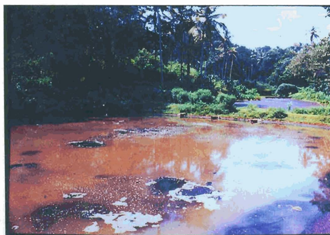
Plate :1 A view of the sewage stabilization pond
