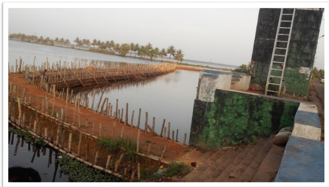
Plate.3. 2. Traditional way to prevent saline intrusion (Valayakettu)
