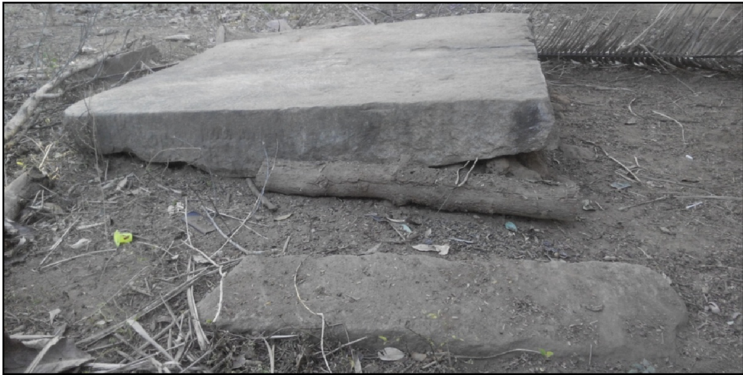
Figure 5: A granite cap stone
