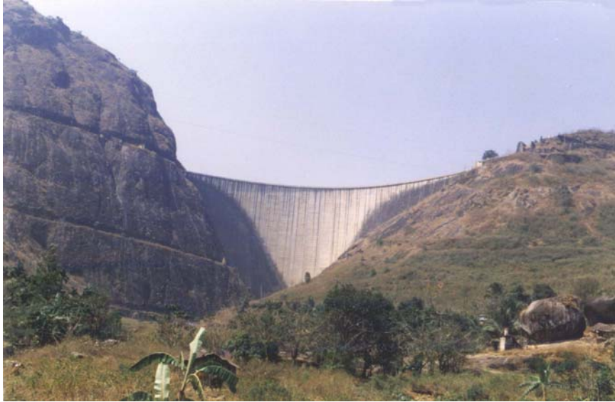
Fig 6.21: Idukki arch dam; view from down stream.
