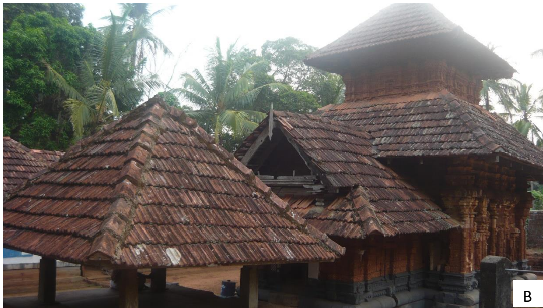
Fig.2. Temples with Granite basement, laterite wall and wooden roof; A- Pulpatta temple, Malappuram dist. B- Pullanur temple Malappuram dist.
